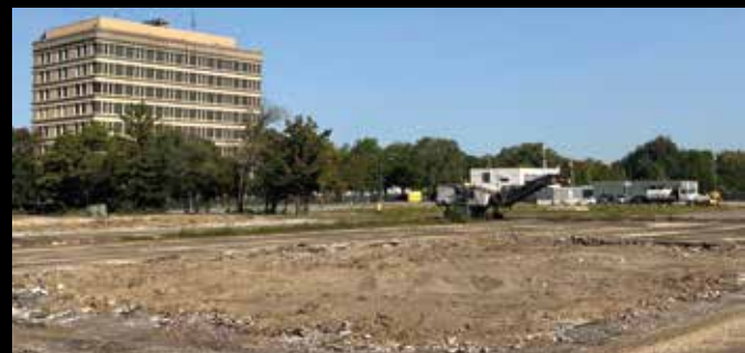
Site-clearing work has begun, in preparation for development
