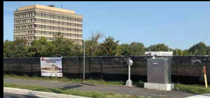
Perimeter fencing along East 38th Street near Meadows Drive
