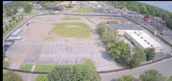
Aerial view of construction site, taken in late August
