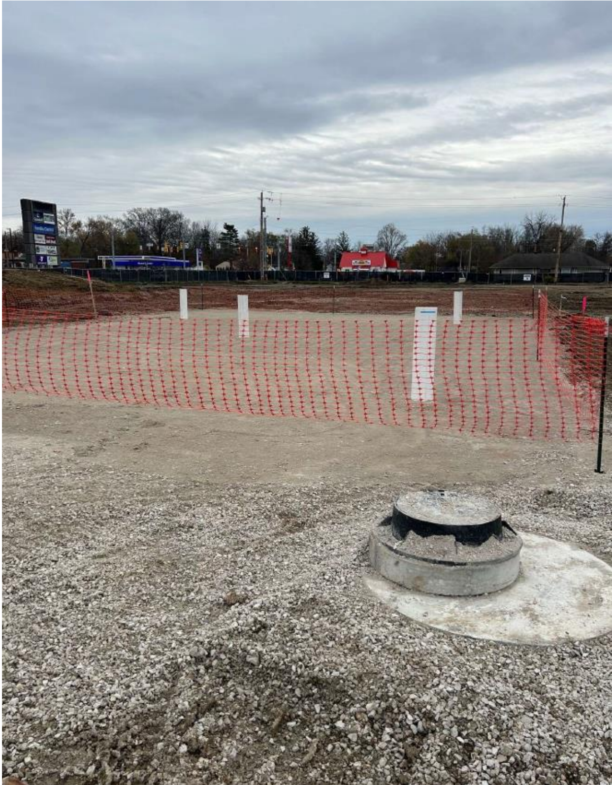
Figure 5: West R-Tank Backfilled, Compacted and Completed
