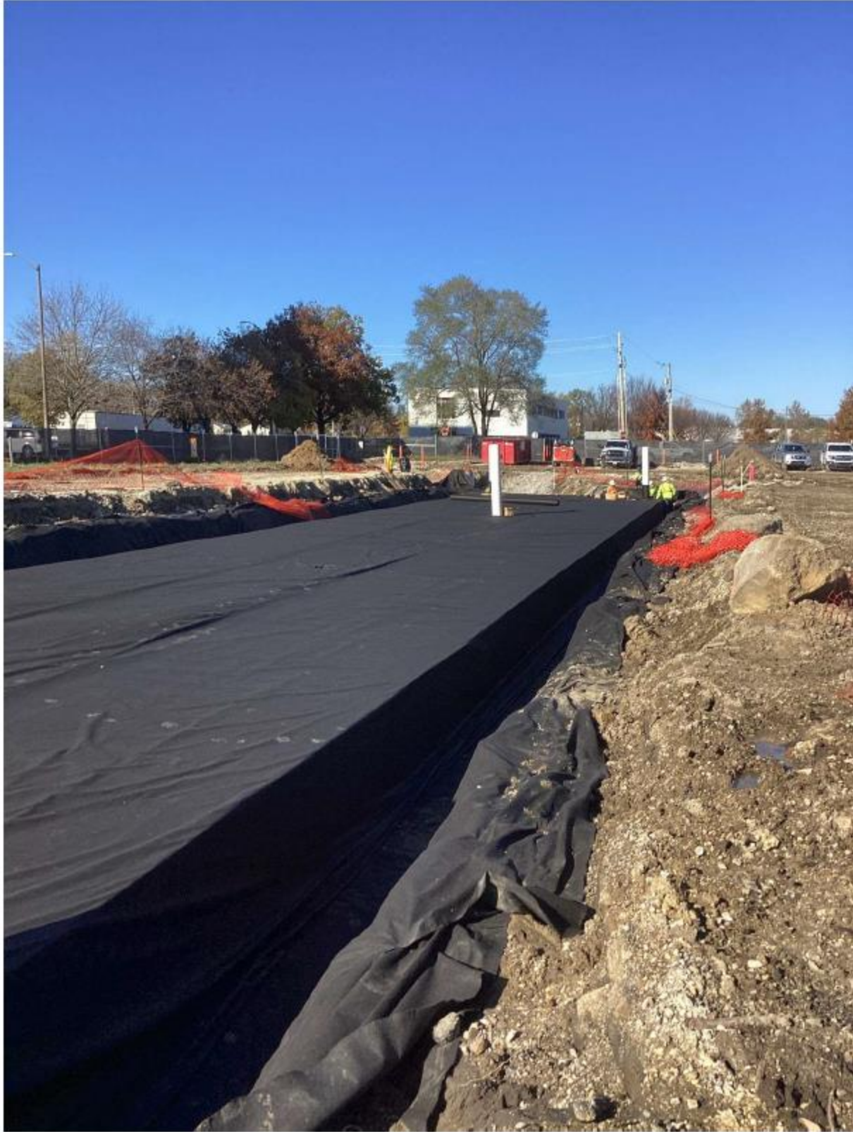
Figure 2: Liner Installation During East R-Tank Construction
