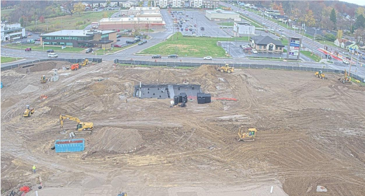
Underground R-Tank installation
