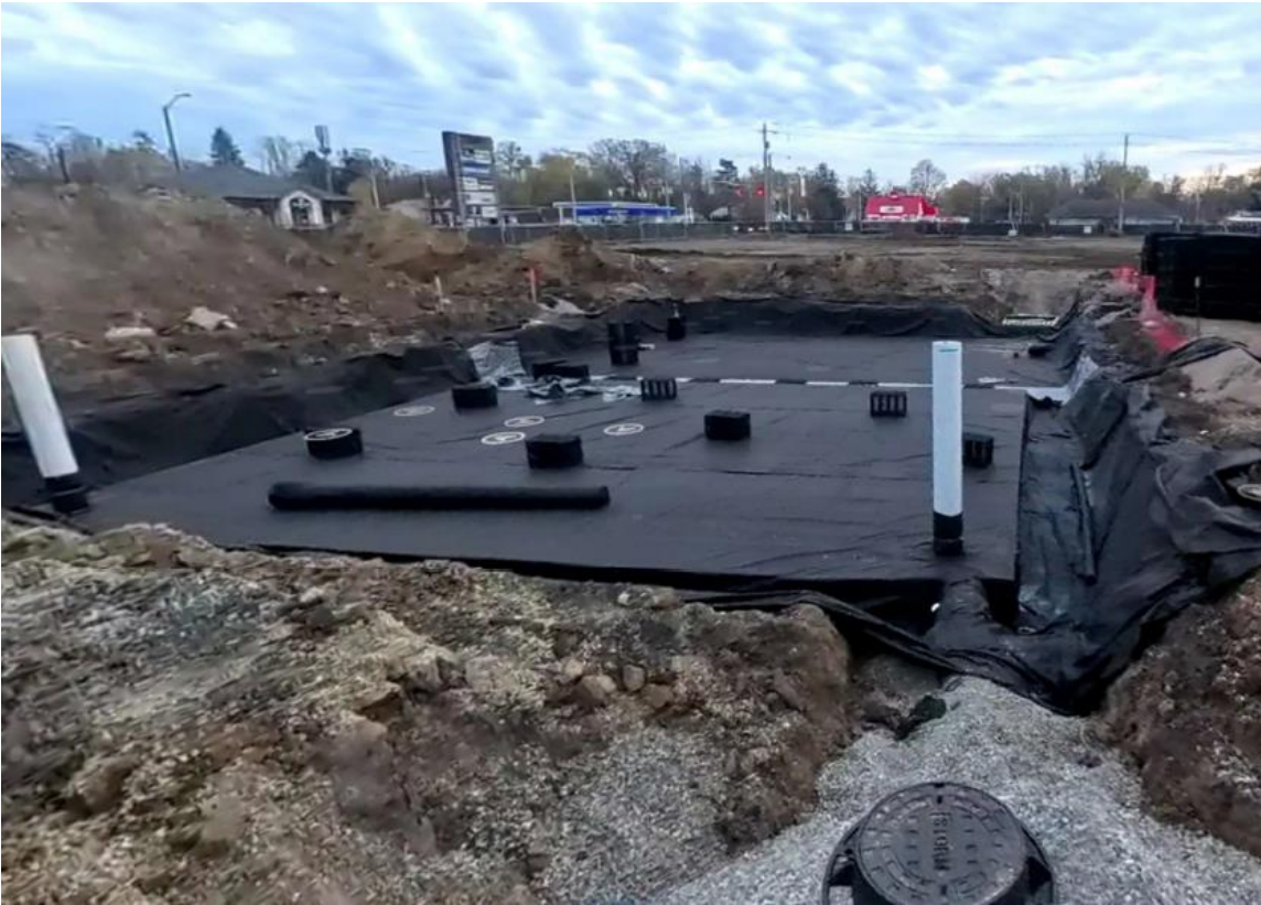
Figure 4: West R-Tank Liner and Crate Installation
