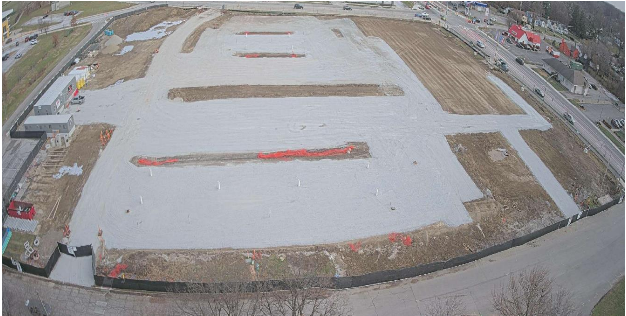
Parking lot surface and road work
