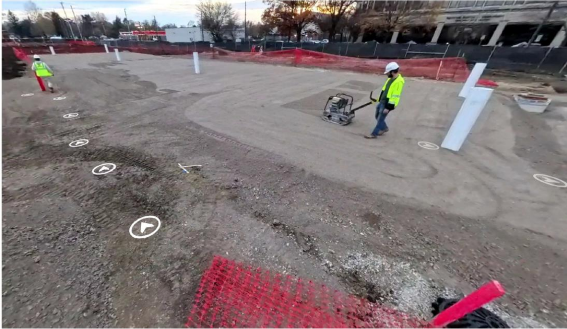
Figure 3: East R-Tank Backfill Compaction
