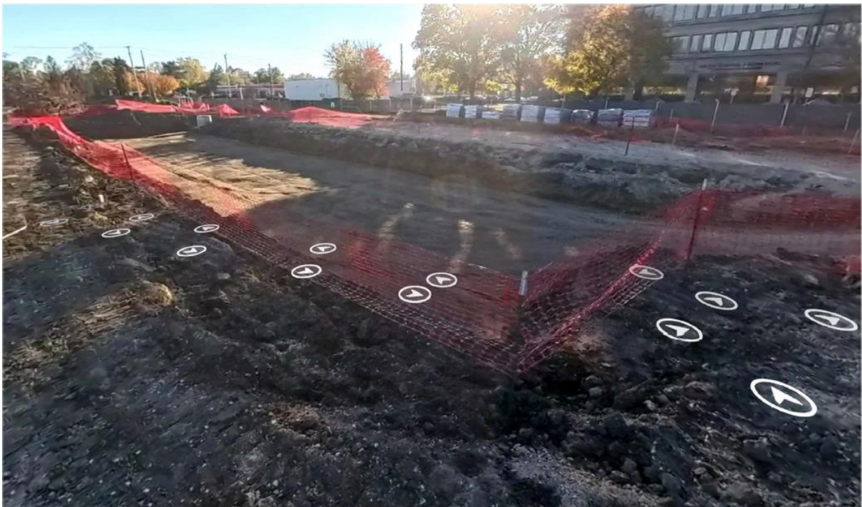
Figure 1: Excavation of East Recession Tank (R-Tank)
