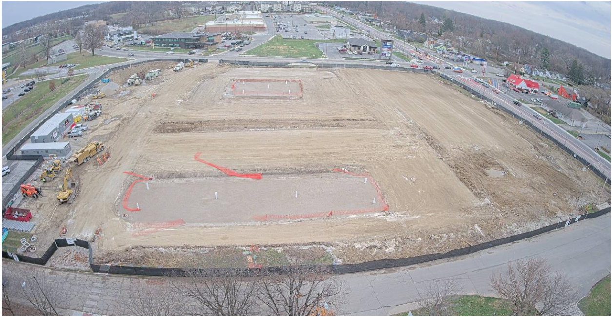
Parking lot surface grading
