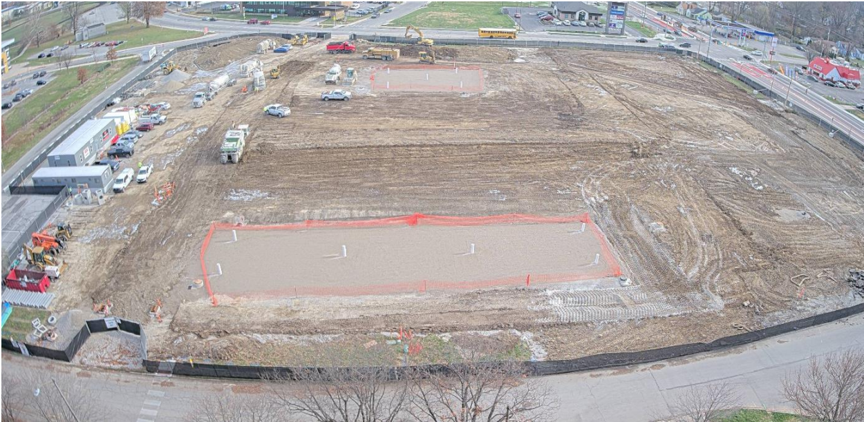
Site leveling and grading work
