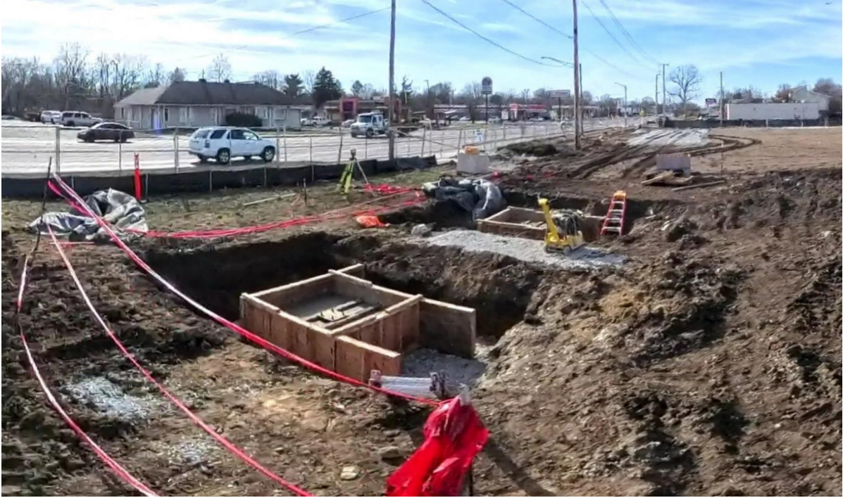
Figure 2: Concrete footers for structural columns
