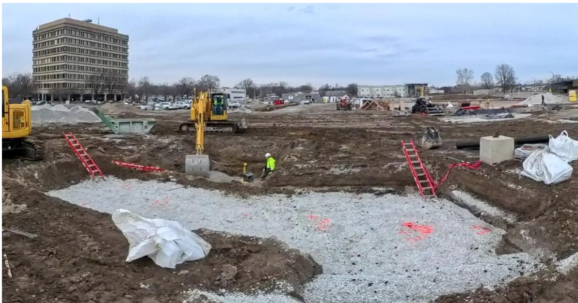
Figure 5: Undercutting for ground stabilization prior to foundation pour
