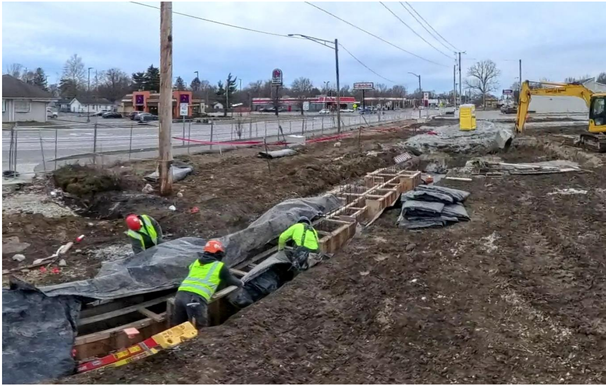
Figure 4: Setting the South Foundation Wall
