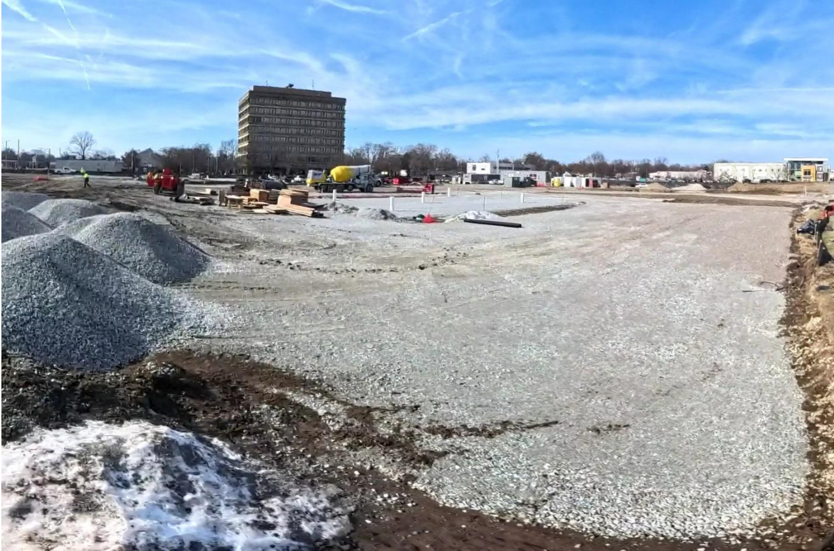
Figure 3: Parking lot stabilization completed
